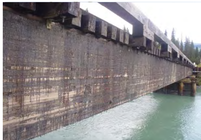
Figure 1-14: Span 2 girder 4 downstream face condition.
