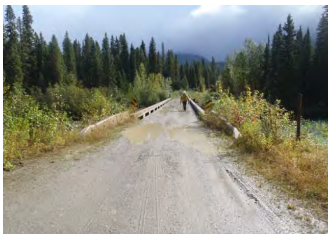
Figure 1-3: Looking towards likely end, not ponding water.
