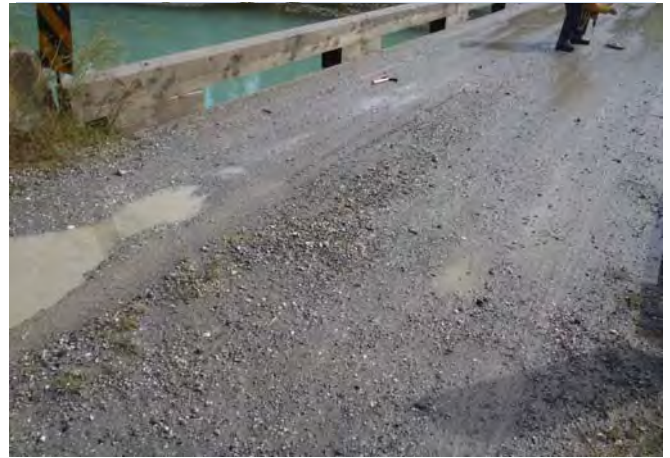
Figure 1-8: Wells end abutment deck end.
