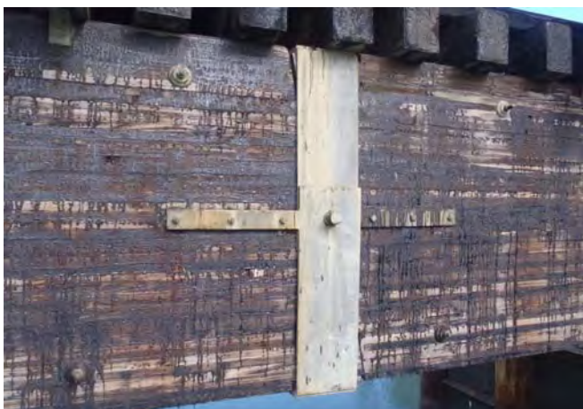
Figure 1-15: Typical hanger condition, span 2 downstream shown.
