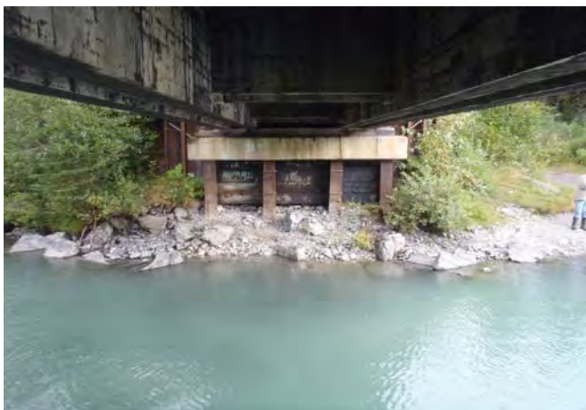
Figure 1-17: Likely end abutment.
