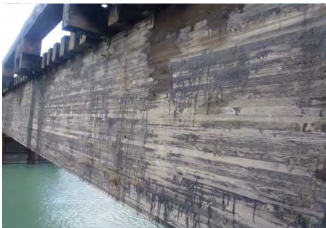
Figure 1-13: Span 2 girder 1 upstream face condition.
