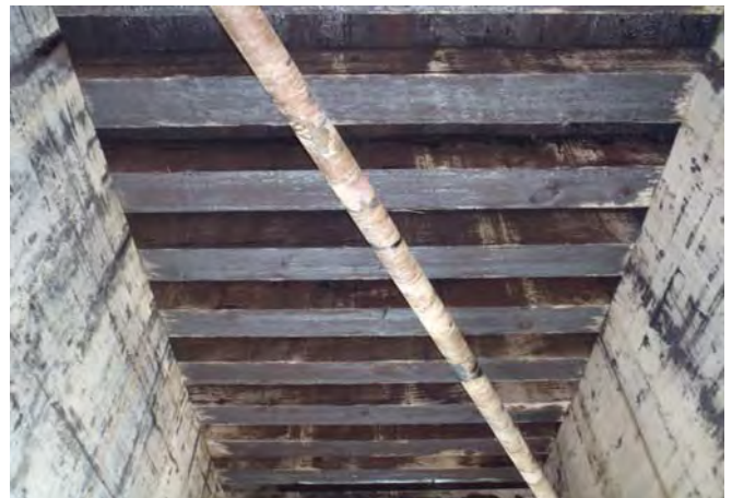
Figure 1-12: Typical sub deck condition, span 2 shown.
