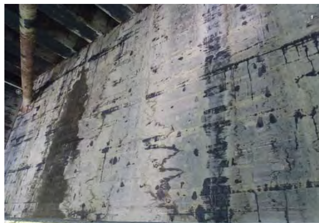
Figure 1-16: Typical interior girder condition, span 2 girder 2 downstream face shown.
